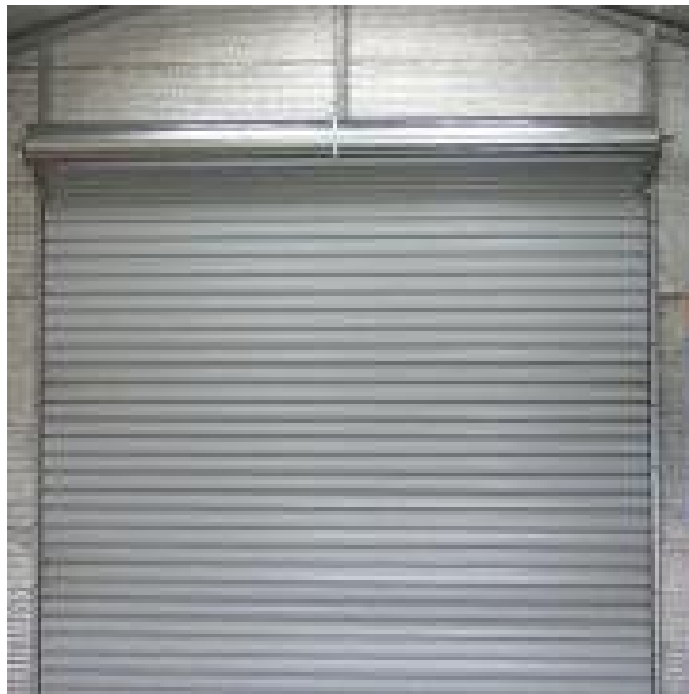
Doors blocking entry to the second floor and outdoor areas
